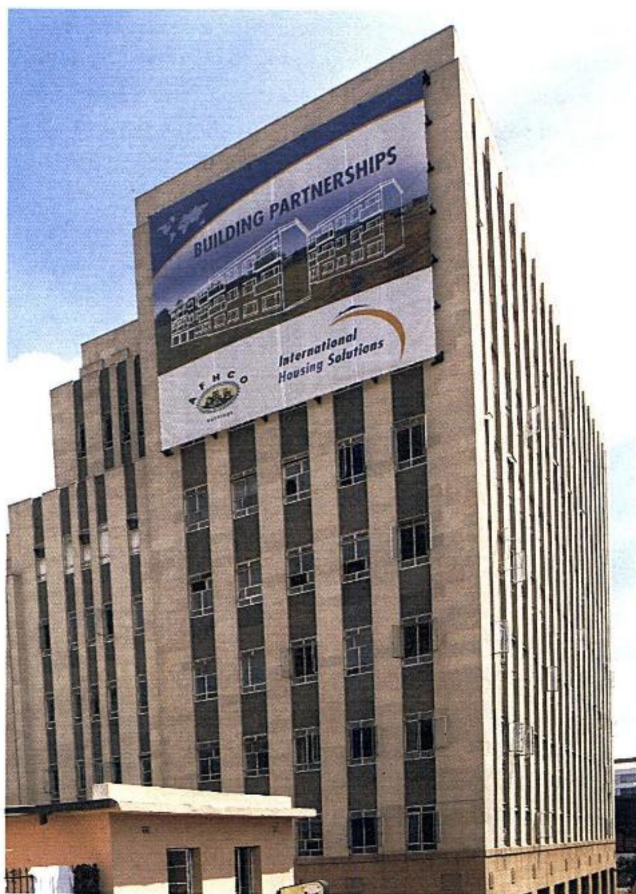
The old Greatermans building in Johannesburg has been converted into low-income housing.
