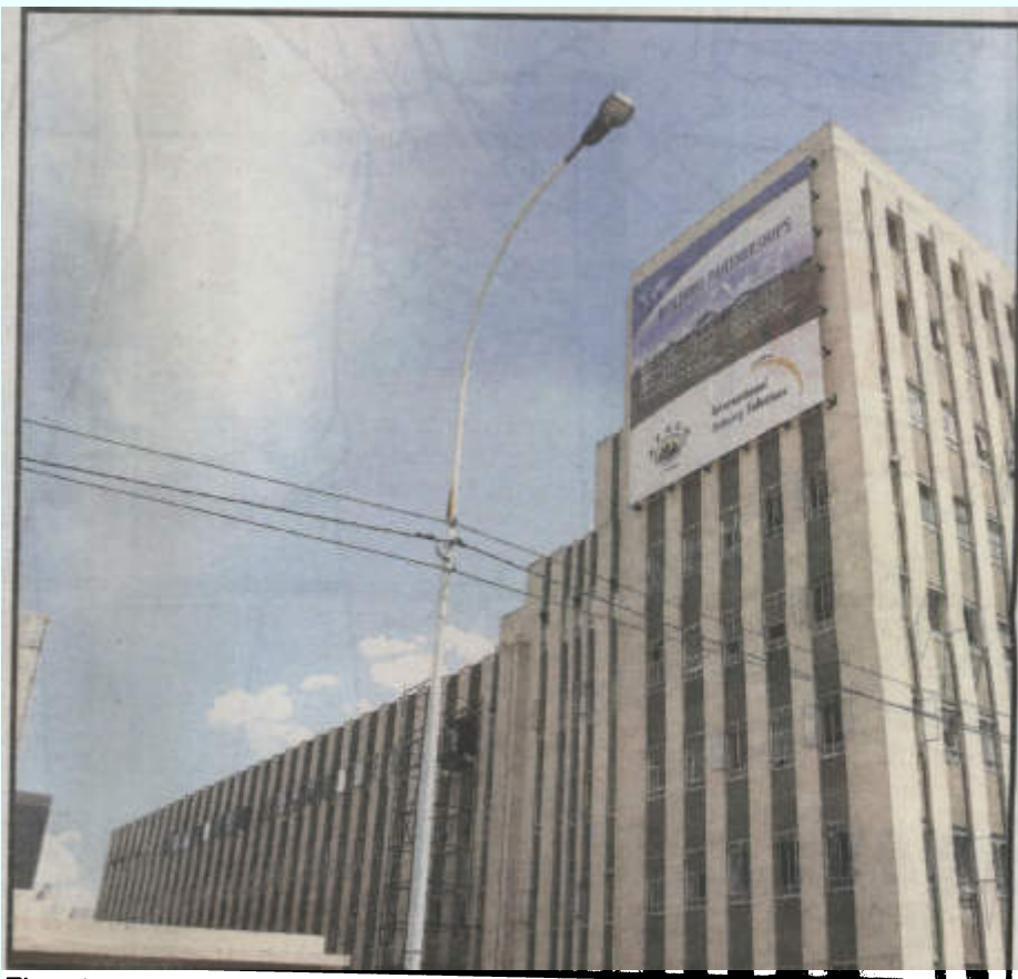
The old Greatermans building which was converted into a stunning block of flats.
